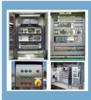
DCS Control Panel Work
