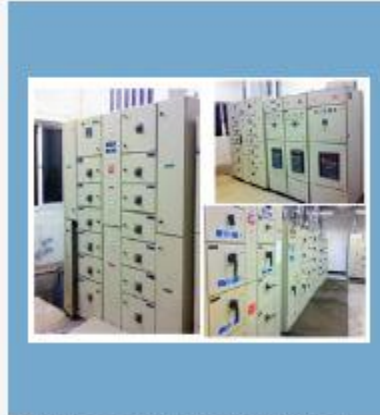
Power Panel Installation
